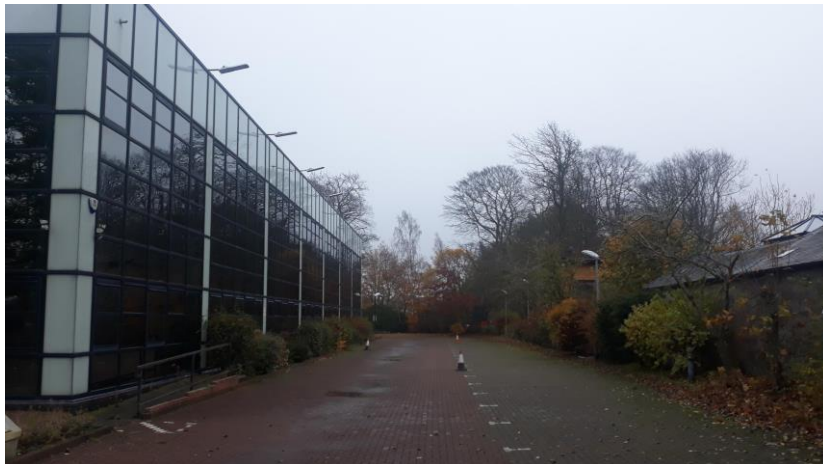
South elevation & boundary
